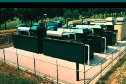
University of Illinois in Chicago installed an L36GL standby set.
