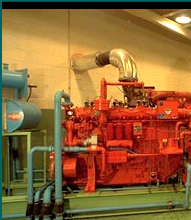
Waukesha VGF F18G drives 90 kW induction generator in parallel with utility for Canonsburg, Pennsylvania, wastewater treatment plant.
